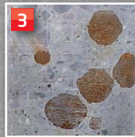
3. Designed for High Strength & Heavily reinforced concrete
